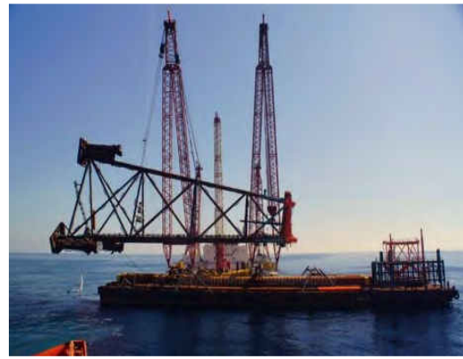
Removal of platform jacket onto barge for transport to shore
