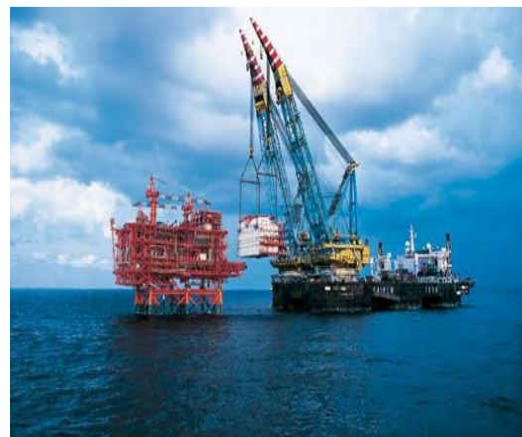
Removal of platform topsides using multiple lifts (option using conventional heavy lift vessel (HLV) – courtesy of Saipem)
