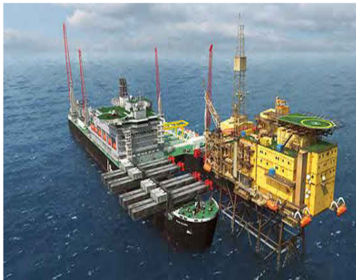
Removal of platform topsides in single lift (option using specialist HLV – courtesy of Allseas)
