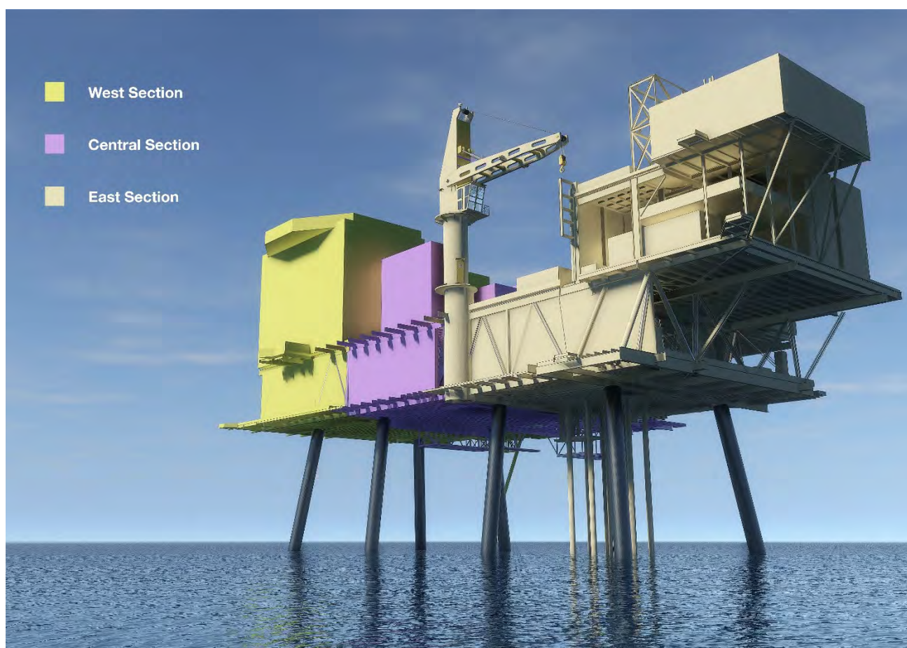
Figure 15: Kinsale Alpha topside schematic showing the topside module sections
