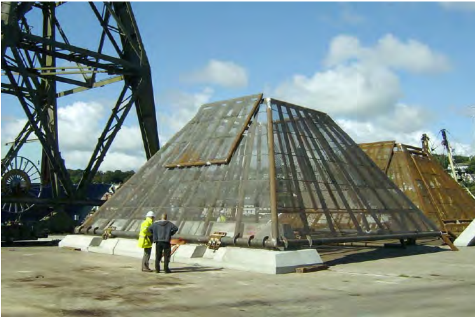
Figure 9: Subsea infrastructure – Wellhead Protection Structure and PLEM
