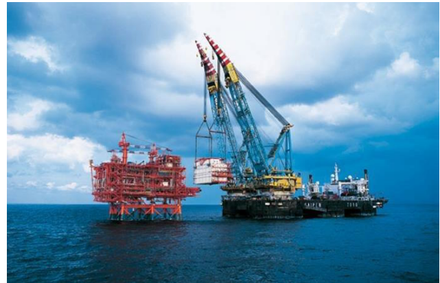
Removal of topside by heavy lift vessel
